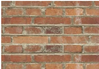
Brick wall detail
