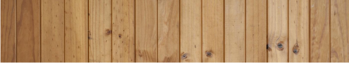
Detail of vertical boards
