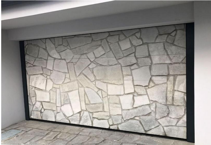
Complete door design: Door matches driveway
